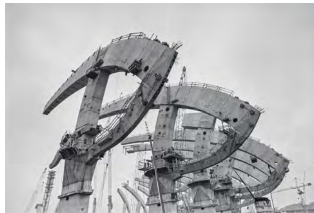
Michel Gravel, The Olympic Stadium Construction Site, Montreal, September 17, 1975 . Gift of La Presse Inc., M2020.95.14.9.2733, McCord Stewart Museum
