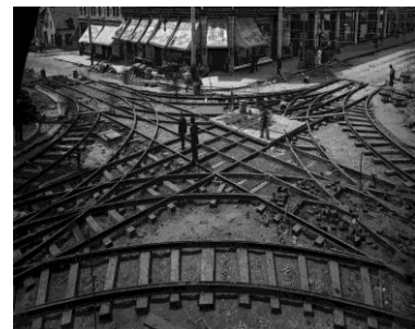
Tramway crossing under construction, Ste. Catherine and St. Lawrence St., Montreal, QC, 1893 Wm. Notman & Son 1893, 19th century
